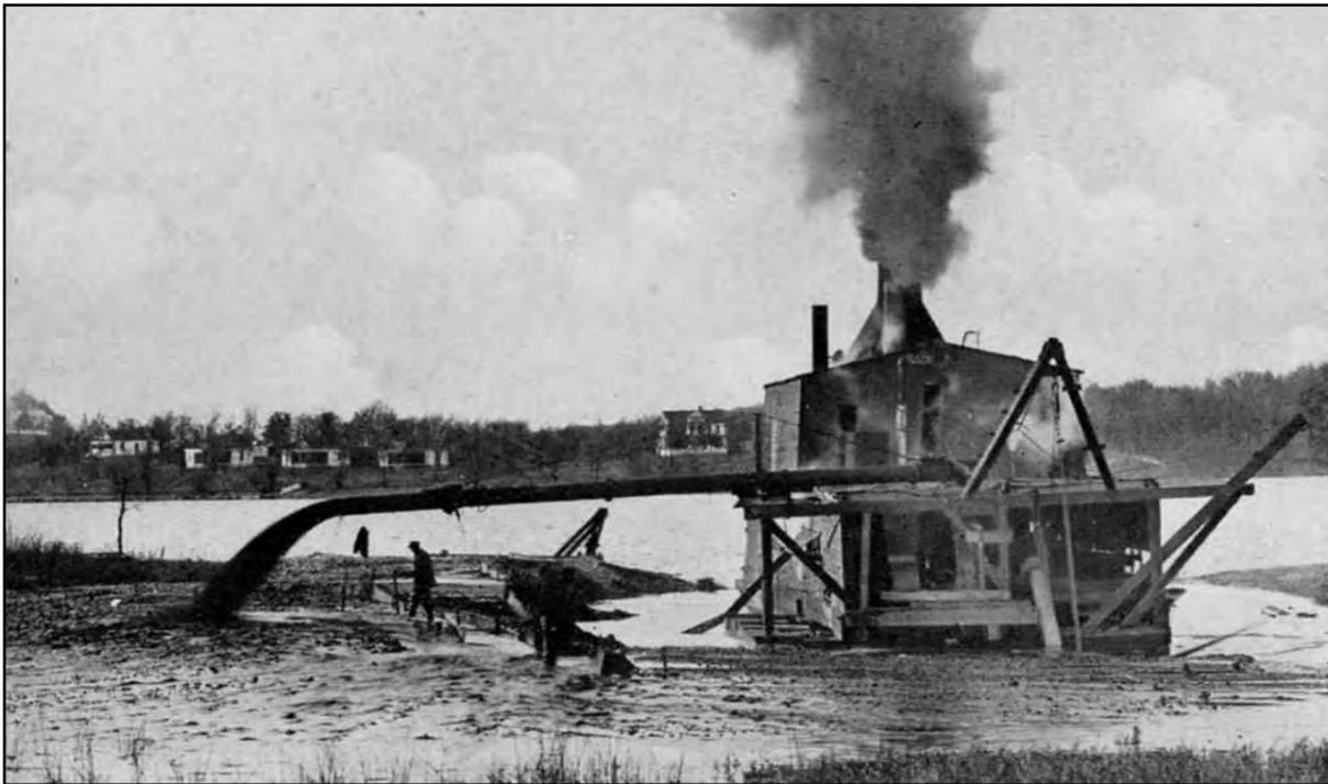
Hydraulic dredge commencing excavation of the Cedar Lake canal. Completion of the link with Lake of the Isles in November 1913 caused the water level of Cedar Lake to drop four to five feet, dramatically altering the lake’s appearance and creating the Cedar Lake we know today. (Photo: Park Board 1912 Annual Report, courtesy Minneapolis Central Library Special Collections.)
